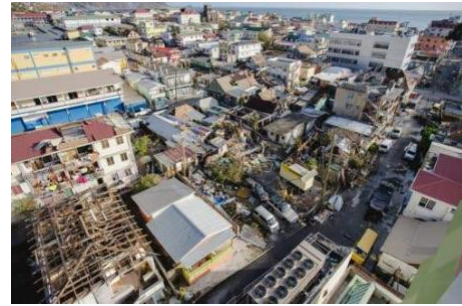
Destruction of Roseau, Dominica post hurricane Maria, 2017, ©Carisealand
